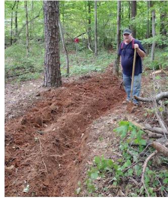
Digging a ditch
